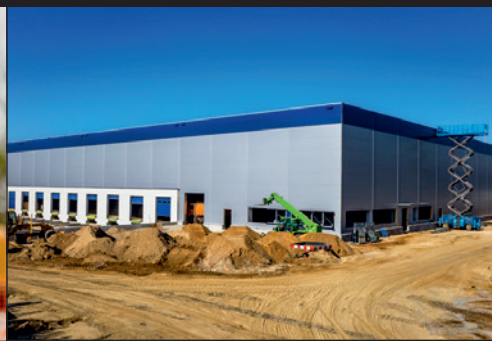
Foundation recommendations for warehouse development
