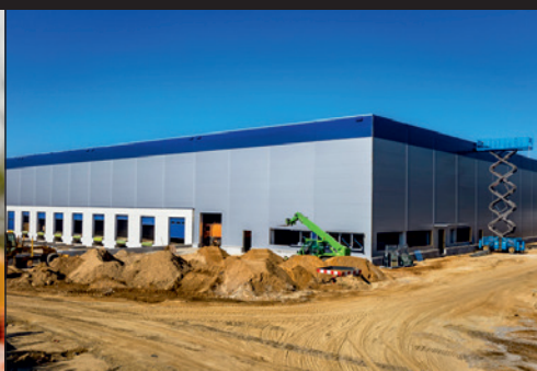
Foundation recommendations for warehouse development
