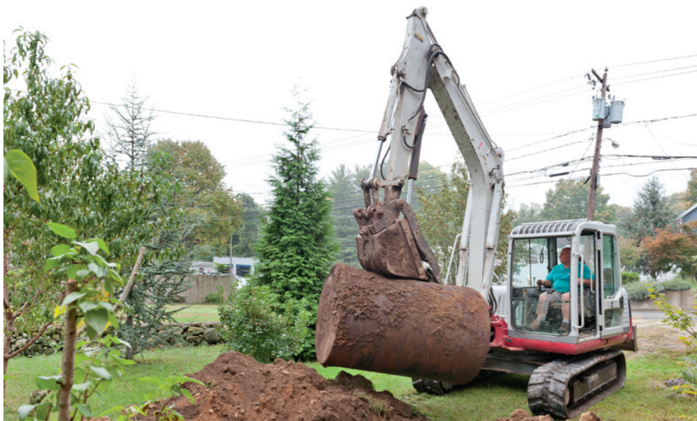
Underground storage tank removal
